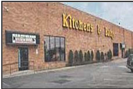
The contract included both the demolition of the old exterior and the installation of the new energy efficient, E.I.F.S. (Exterior Insulation Finish System) facade. E.I.F.S. creates the look of a concrete fortress to the novice eye. It's a lightweight synthetic wall-cladding that includes exterior sheetrock, rigid foam insulation and thin synthetic coatings. One of the biggest benefits of this system is that the insulation increases the "R" value making it much more energy efficient.
